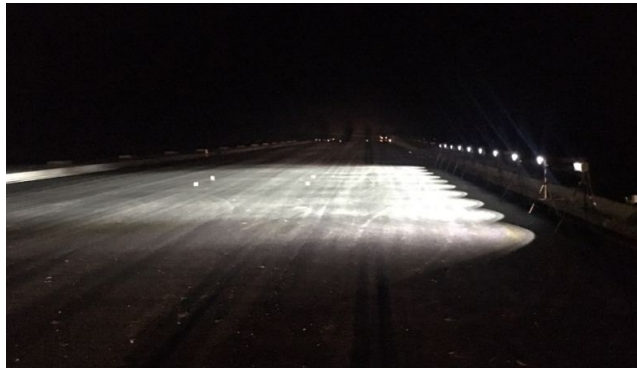
Figure 2. Trial products installed
